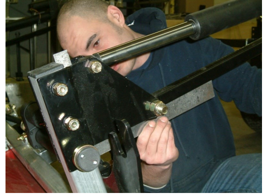
Figure 7: Squaring float arm assembly
