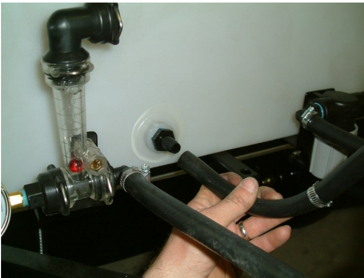
Figure 7: Attaching return line from Pressure Regulator
